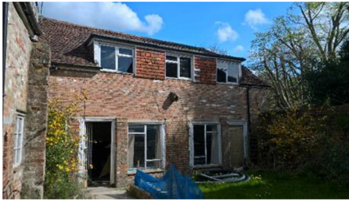
Photograph of the existing building
