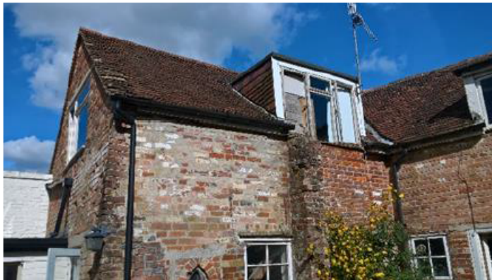
Photograph of the existing building
